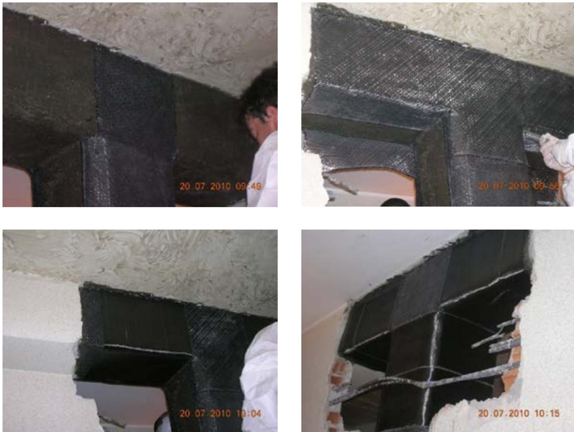
**Fig. 27** - Strengthening of the joint panel in an unconfined interior joint
