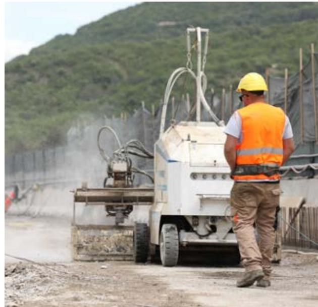
Unlike abrasive blasting, selective hydrodemolition also enables the removal of cohesive portions of concrete, ensuring a high-quality surface roughness.
