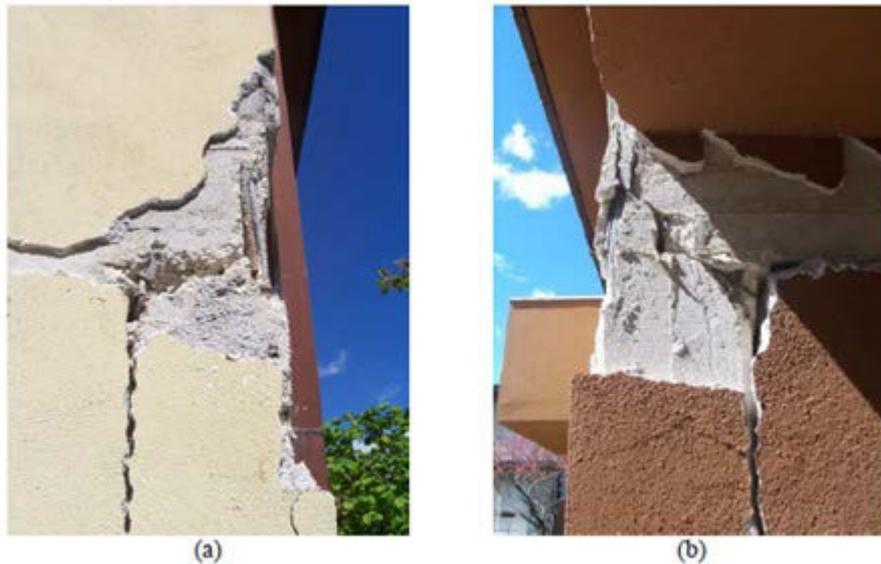
*Fig. 25 - Typical cracking patterns observed in joint panels [01]*
