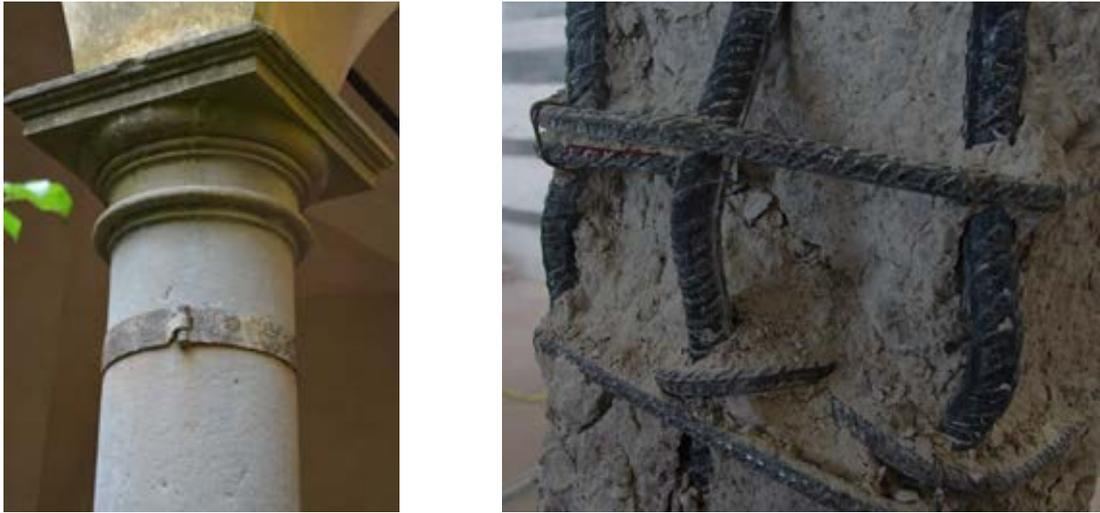
*Fig. 09 - Buckling of compressed reinforcement bars*
